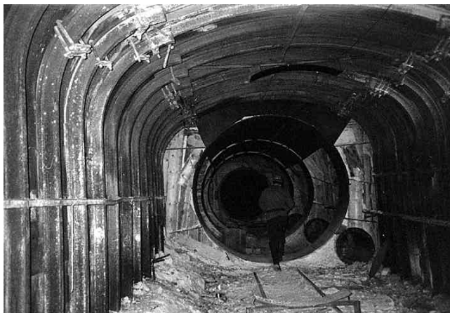
Figure 16. Tunnel entrance at Degelen mountain, with supports visible for a large-diameter line-of-sight pipe. Such structures, evacuated, were used to direct a beam of radiation to test objects located outside of the tunnel complex.
